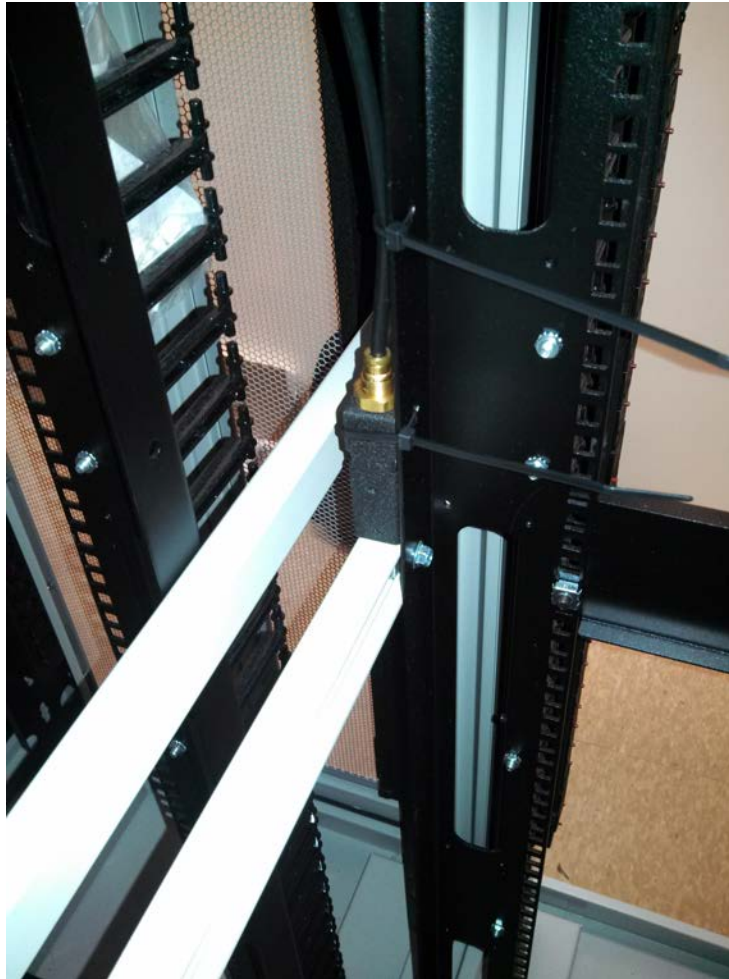
Figure 3-8 Pressure Sensor Hose Location
